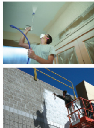
Cordless airless sprayer is ideal for small jobs spraying protective coatings
