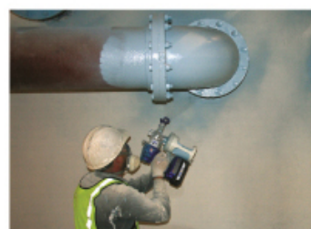
Cordless airless sprayer is ideal for small jobs spraying protective coatings
