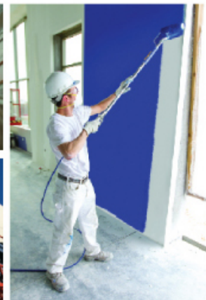
Cordless airless sprayer is ideal for small jobs spraying protective coatings
